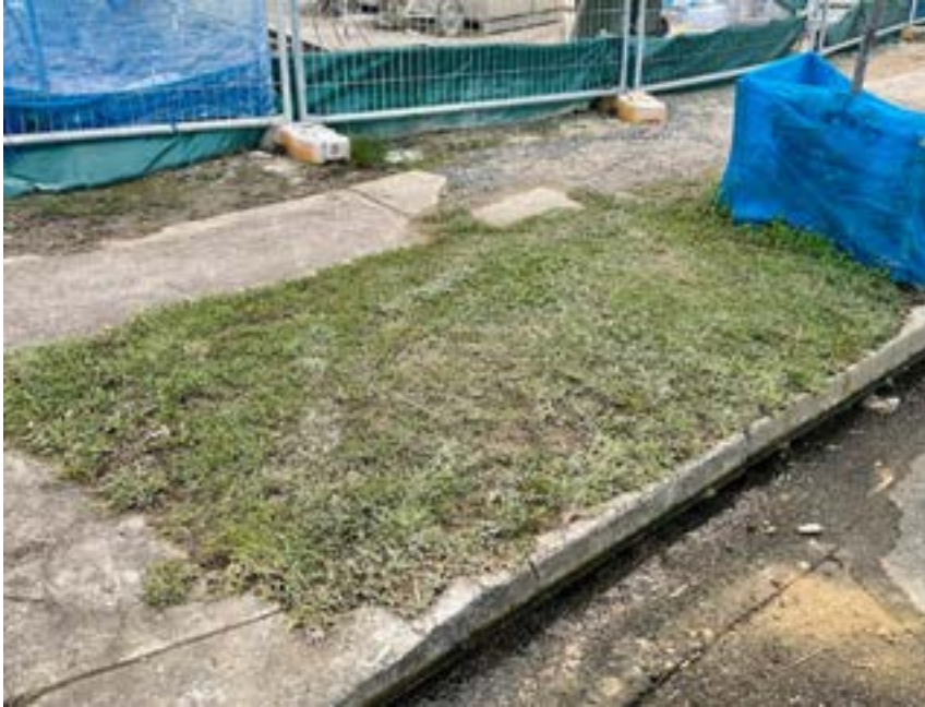
Figure 13. Grass strips by a road that control sediment in low flows. Source: Parramatta River Catchment Group
