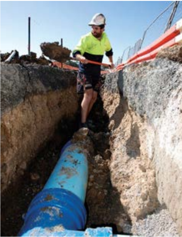
Figure 15. A construction worker installs a service trench
