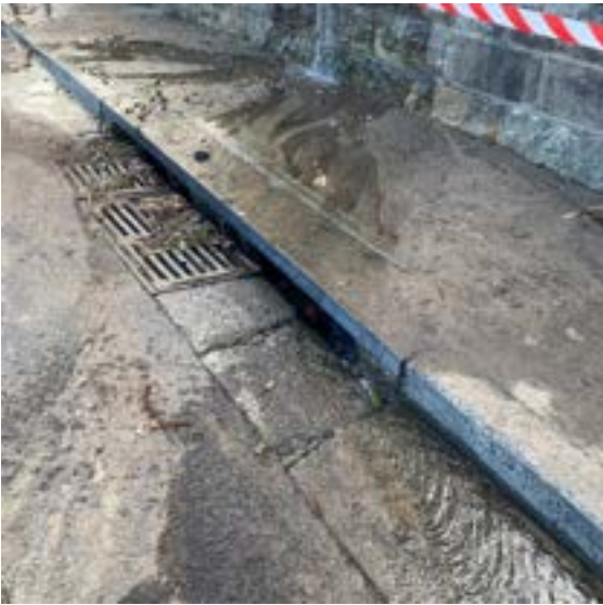
Figure 12. Sediment and debris are affecting a stormwater drain without a sandbag kerb sediment trap
