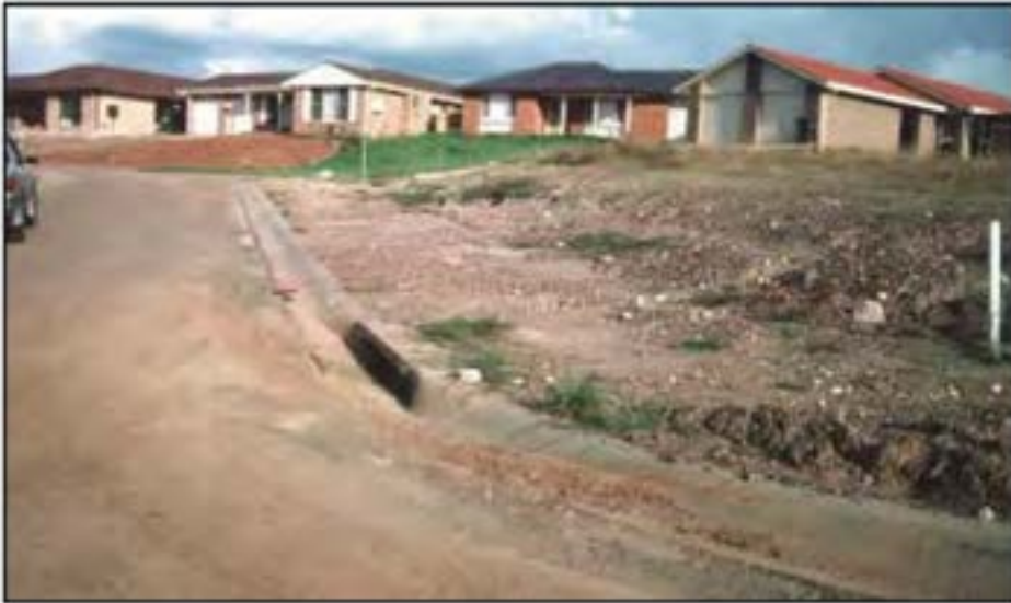
Figure 16. A poorly stabilised site resulting in sediment run-off onto nearby roads and into drains. Source: Managing Urban Stormwater: Soils and Construction , 4 th edition
