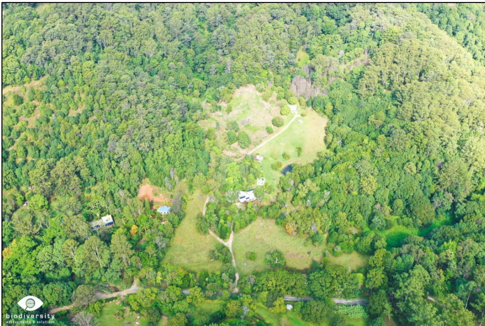
Plate 1: The subject land is vegetated with cleared areas around existing dwellings and current access.
