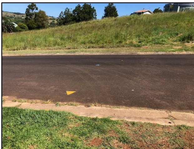
Existing fire hydrants in Rankin Drive.
