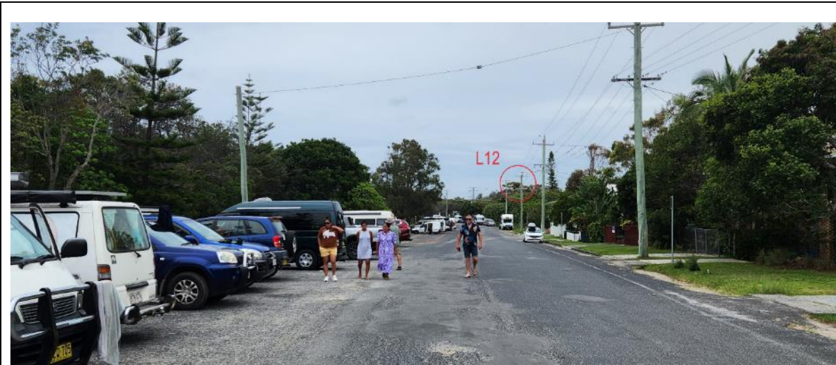
Plate 11: Essential Energy street lighting at South Beach Road (L12)
