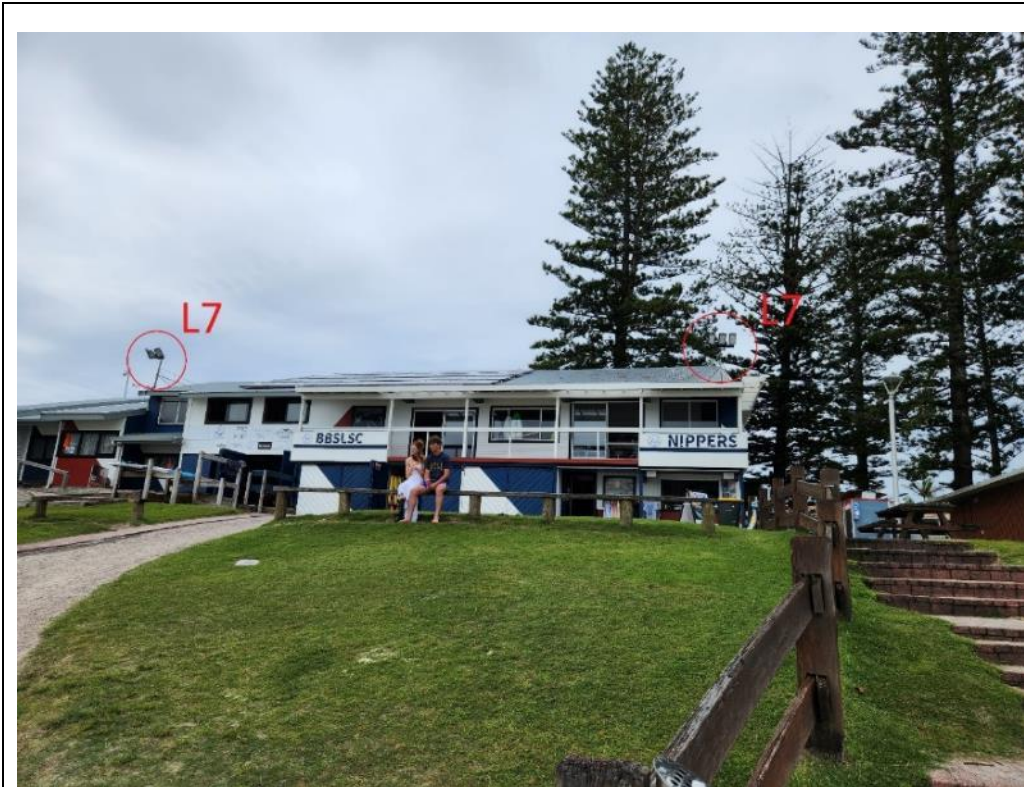
Plate 6: Roof mounted floodlights directed towards the beach at the Byron Bay Surf Life Saving Club (L7).
