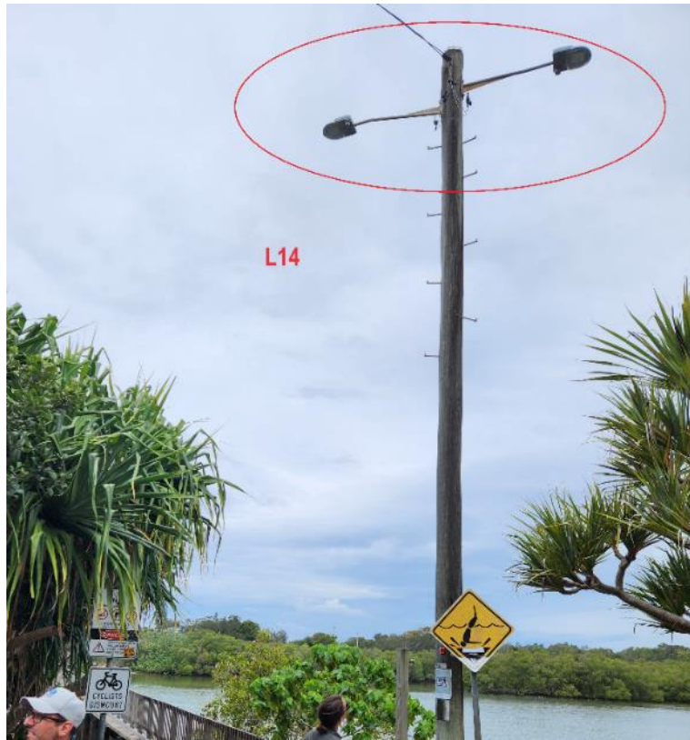
Plate 13: Double light fitting with problematic light spill (L14) immediately adjacent to Simpsons Creek.
