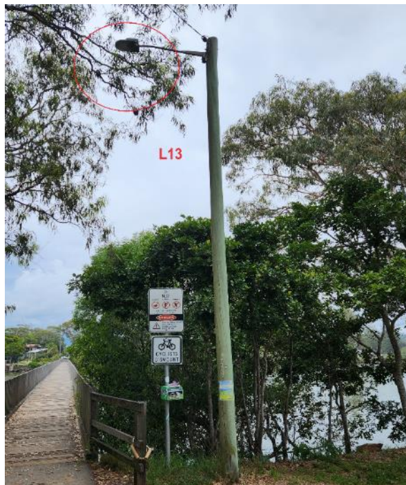
Plate 12: Low wattage light fitting (L13) illuminating canopy of mature tree adjacent to Simpsons Creek at the footbridge, Brunswick Heads.
