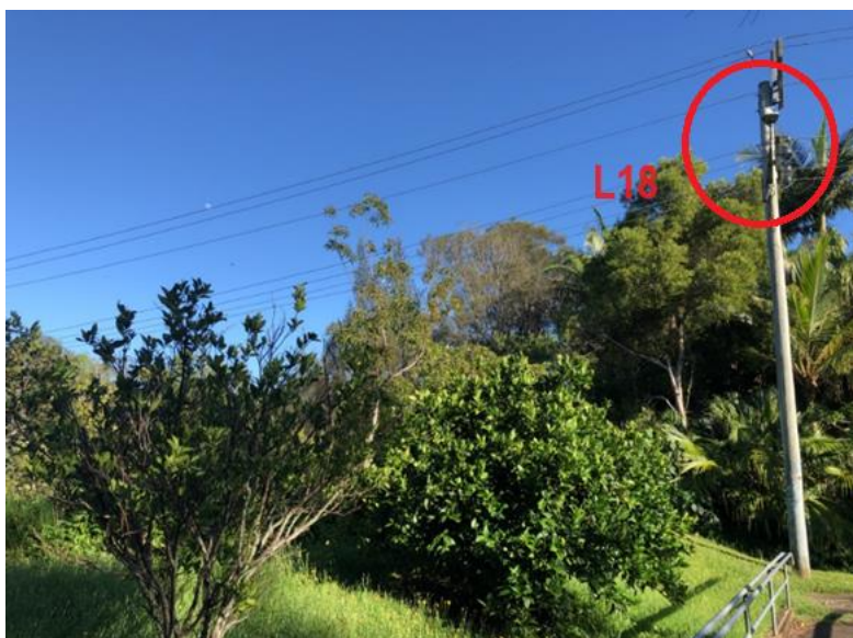
Plate 17: Essential Energy pole-mounted streetlight at the Helen Street footbridge over Yelgun Creek. There are few other streetlights in proximity to the creek. Some vegetation provides light screening between the creek and this light source. The direction (downfacing) and low wattage (18W) would provide low level illumination to the waterway and adjacent vegetation. Replacement of this light with a low-level bollard could be considered.
