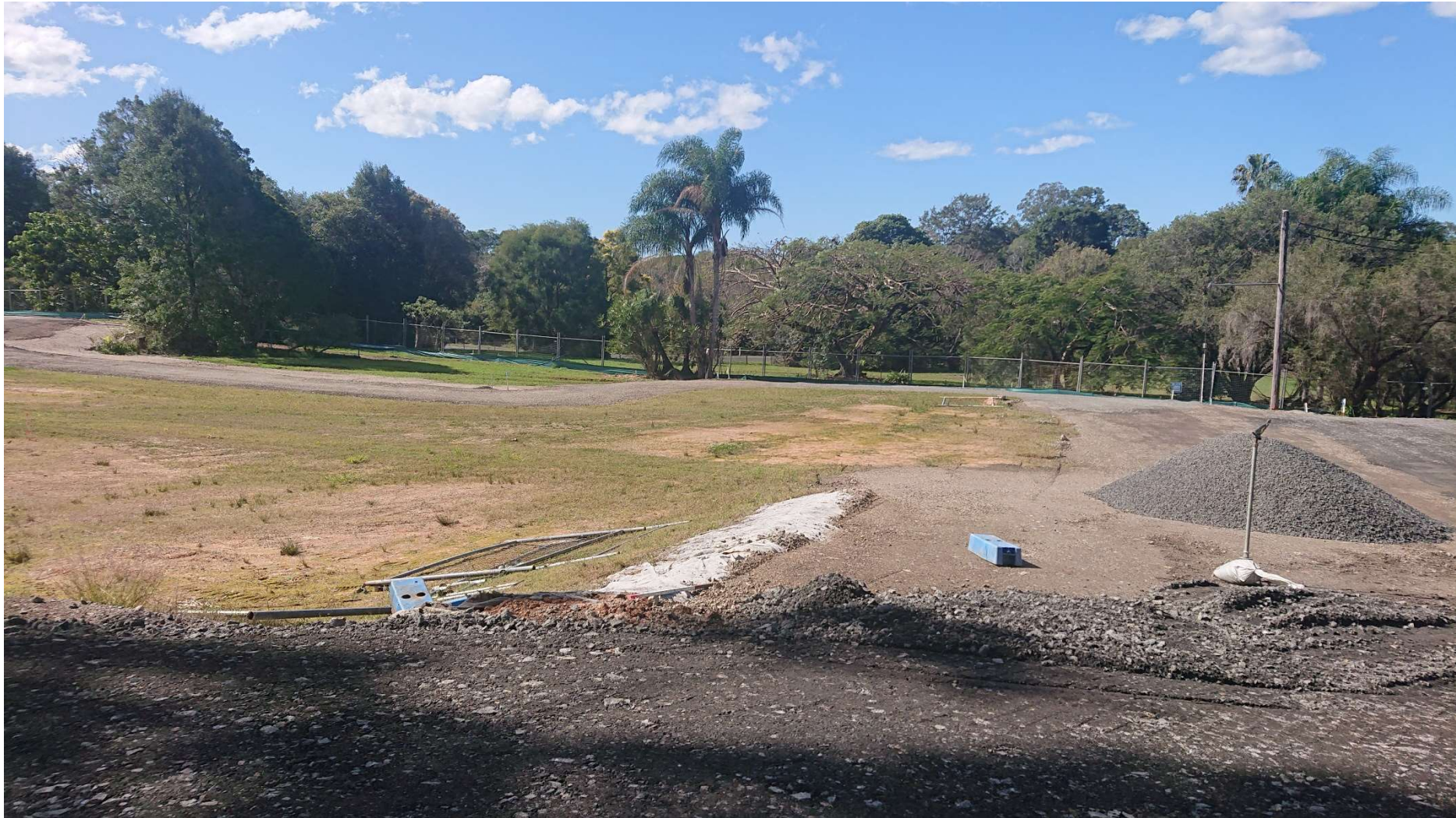
Plate B7. Easterly view of southern section of encapsulation area (overlooking Block A) (16 th August 2022)
