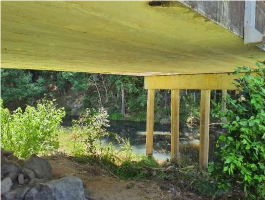
Plate B. View below western bridge abutment.
