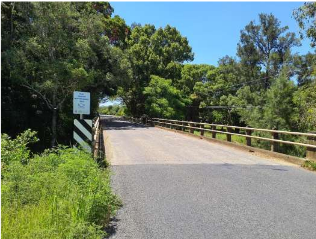
Plate A. View east across Sherry bridge. Access track will be located adjacent the northwest bridge abutment (left in image).
